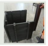
Slide 1x post with dovetail groove and square groove onto panel and push until it comes into contact with ground.
