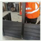
Push corner post down the 2 panels until it comes into contact with the ground as shown.
