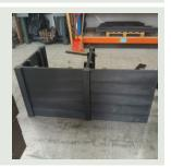
Take middle panel and place as shown in picture (note that the middle panel is 675mm and has two sets of ties)
