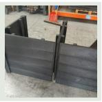
Take 2nd corner post with 2 x dovetail joints and place over the 2 panels.
