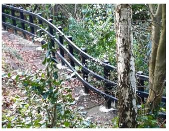
Posts can be anchored to the ground using the same method as timber and steel posts, by concreting, hammered mechanically or surface fixed.
