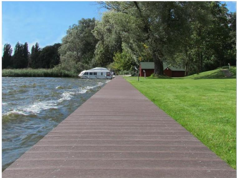
The decking boards available from British Recycled Plastic Products are produced in 3600mm lengths and can be worked using standard wood working tools in the same manner as wood.
